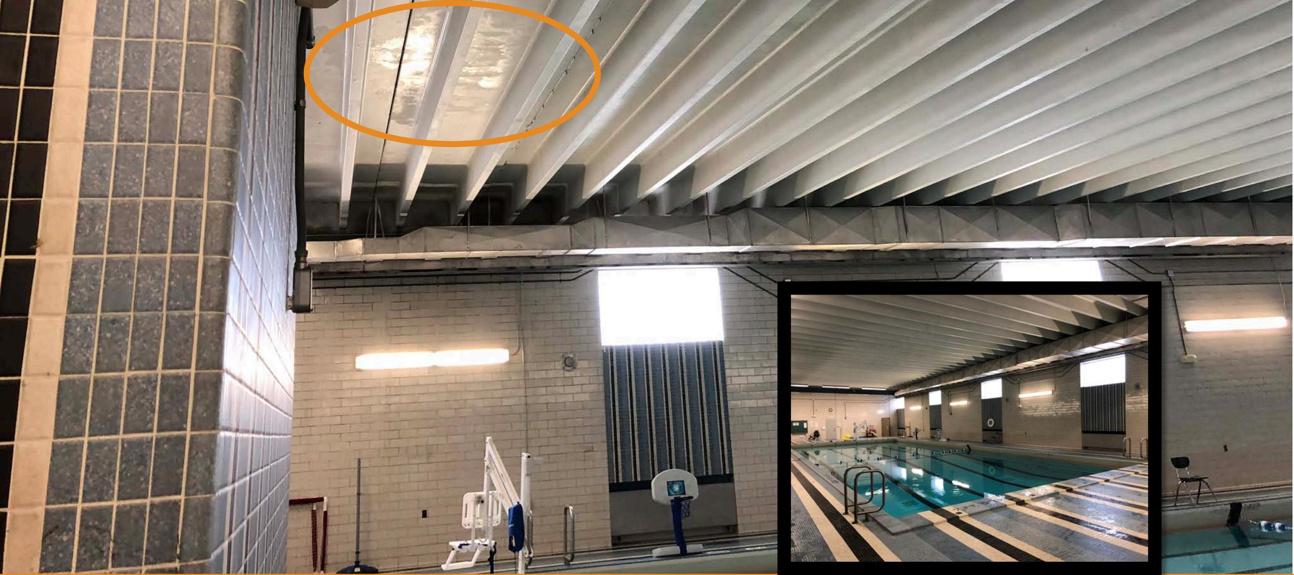
**Condensation in pool due to faulty HVAC and saturated or insufficient roof insulation**
